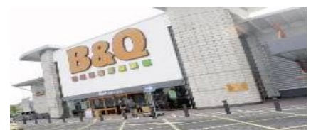
The finished B&Q building
